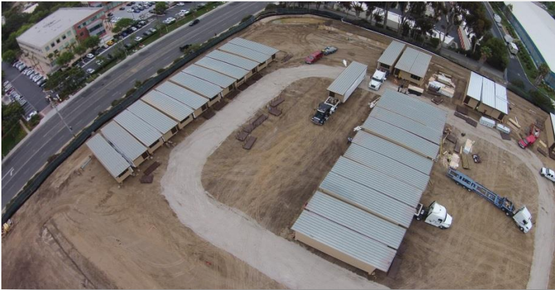
EWMS – Aerial View
