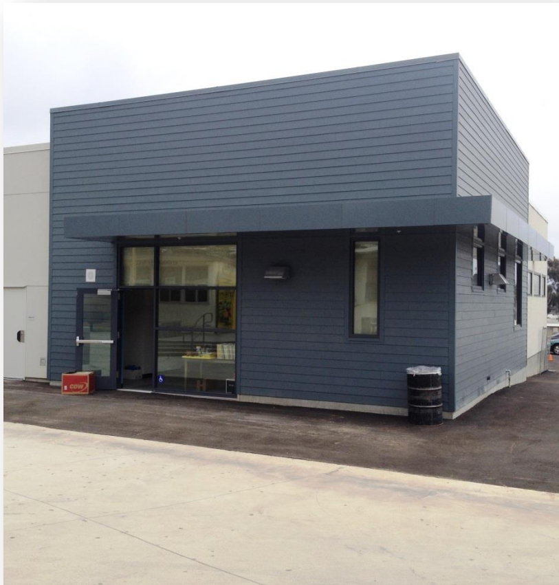
EWMS - Data Center
