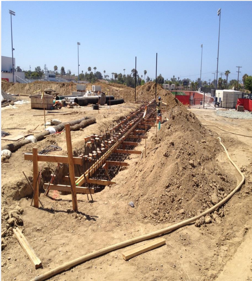
SDHSA – Tennis Courts
